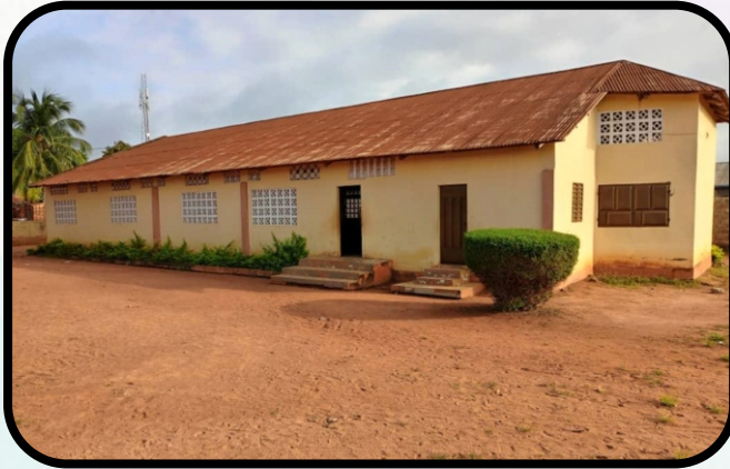
SIDE VIEW OF CHURCH BUILDING
